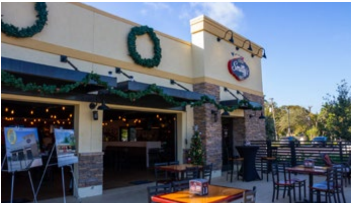
Completion of Smitty's Wings Restaurant
