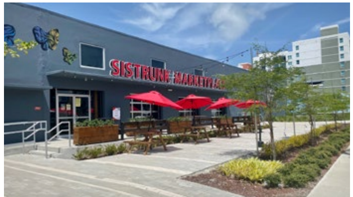
Completion of Sistrunk Marketplace Exterior
