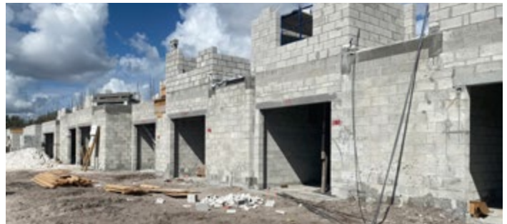
Construction of the River Gardens Townhouse project
