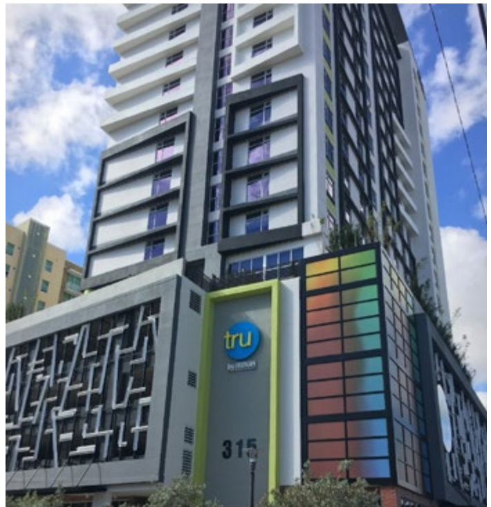
Completion of Flagler Village Hotel
