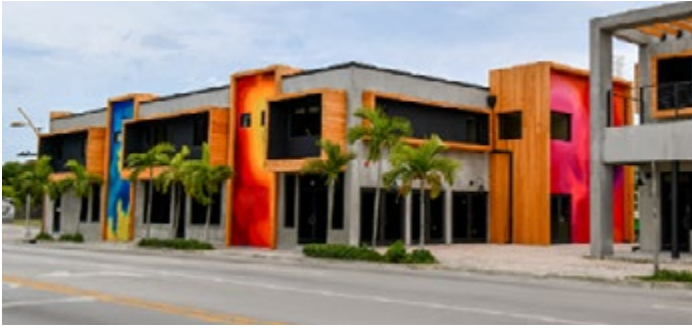
Completion of the Pharmacy Exterior
