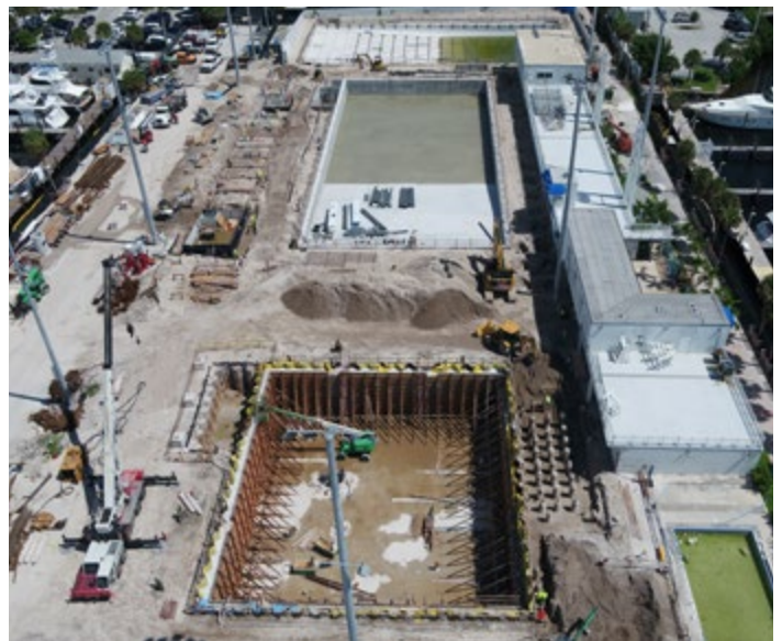
Construction of Fort Lauderdale Aquatics Center Renovation
