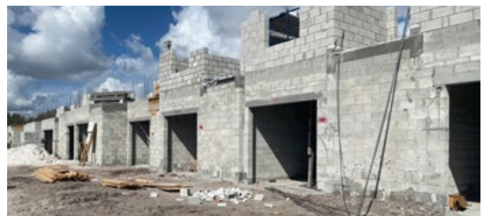
Construction of the River Gardens Townhouse project
