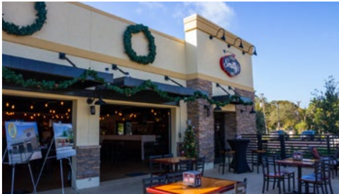
Completion of Smitty's Wings Restaurant
