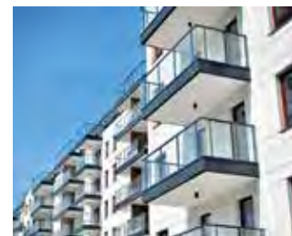
Balconies and cantilevered elements
