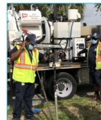
Photo of City worker repairing and maintaining a water main.
