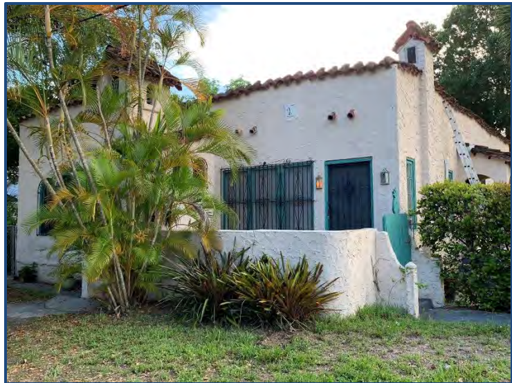
Figure 15: Lady Clare Fursman's House at 401 SW 9 th Avenue (Photo by Trisha Logan)
