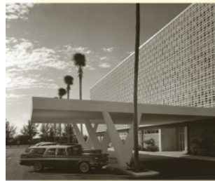
Ripe for adaptive re-use. The Bayview Building, west wing. Built in 1956, it was fused in 1960 to a taller building sheathed in a see-through mesh brick in a folded plate design.
