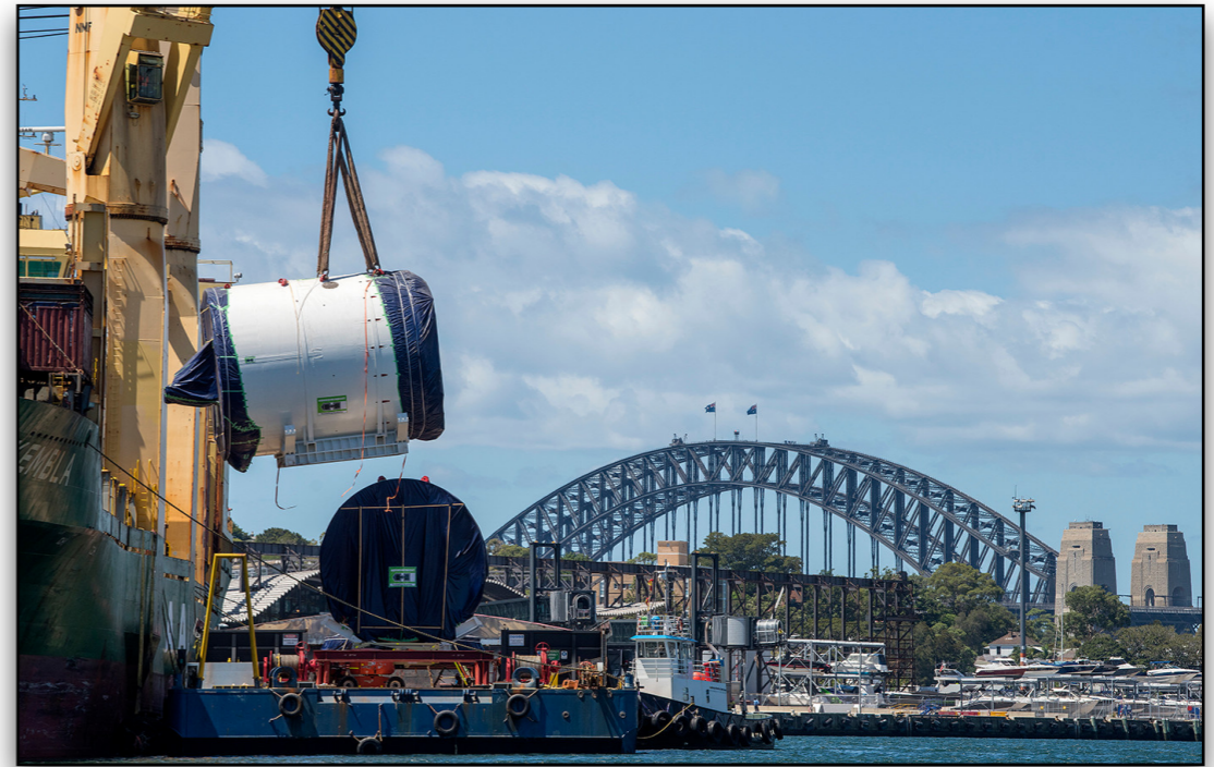
Ghella tunnels under Sydney harbor for a metro line project.
