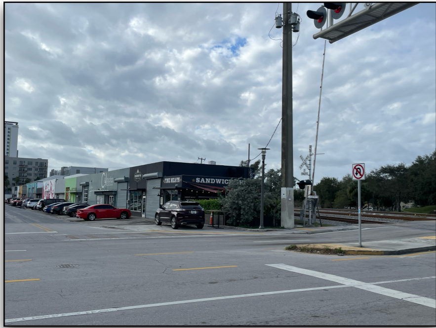
Hines' FATVillage site. The bridge would be at about 25 feet high at NE 7 St. and reach its maximum height by NE 5th St.
