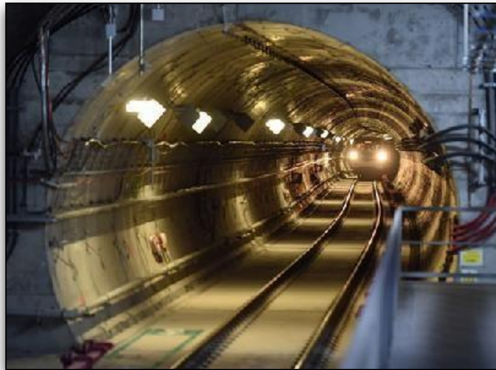
FCC opens an expansion of the metro system in Romania's capital of Bucharest.
