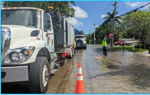
City crews respond to stormwater flooding in River Oaks using pump trucks.
