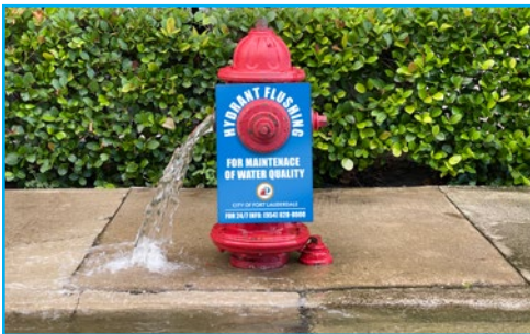
Hydrant flushing as part of preventative maintenance.
