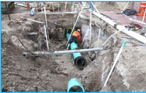
Construction at Pump Station A-7 in Downtown.
