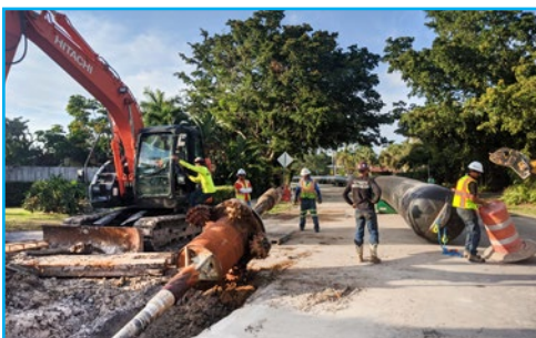
Redundant sewer force main construction in Coral Ridge.
