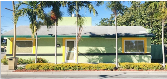
Completion of improvements to 1545 Sistrunk Boulevard for restaurant use
