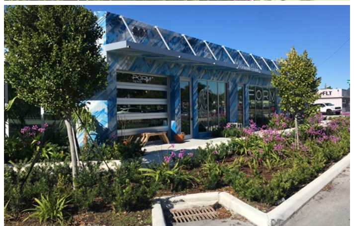
Completion of the Fabrick Project at 801, 807, 815 and 819 NE 2 Avenue in Progresso Village
