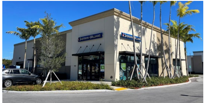
Completion of Sherwin-Williams Store
