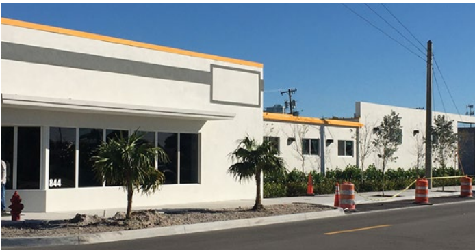
Commencement of renovation and expansion of Hoover Canvas products at 900 NW 9 Avenue
