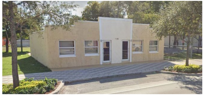
Existing Building at 1108 Sistrunk Boulevard
