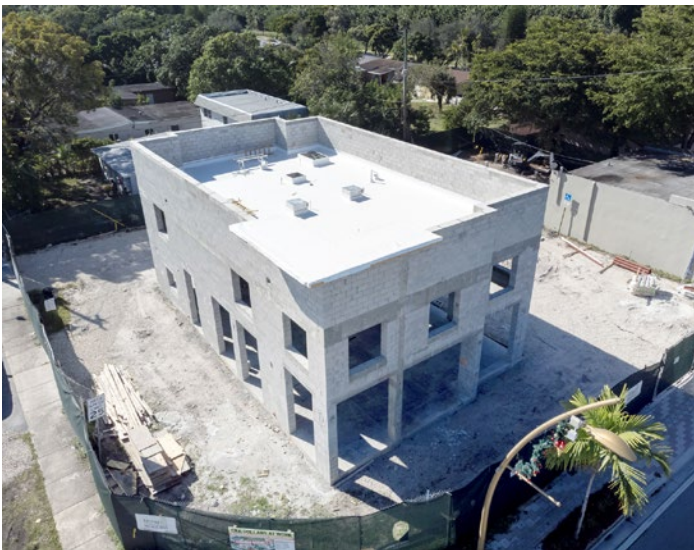
Commencement of construction of Donna's Caribbean Restaurant at 2012 Sistrunk Boulevard
