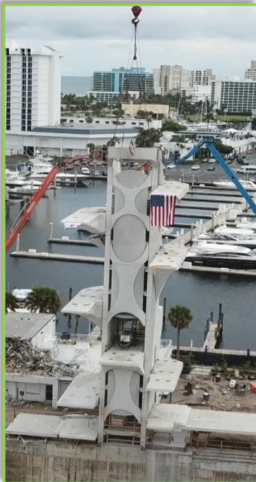
The dive tower under construction
