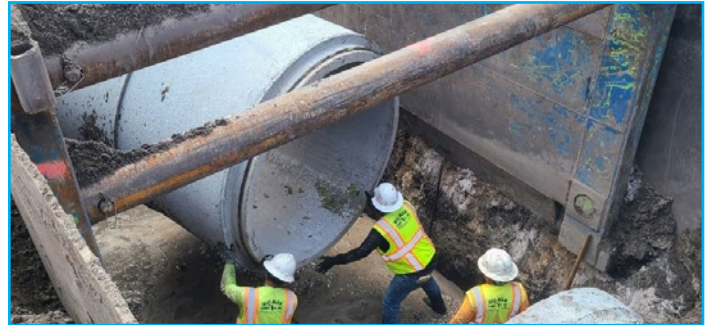
Stormwater pipe installation in River Oaks
