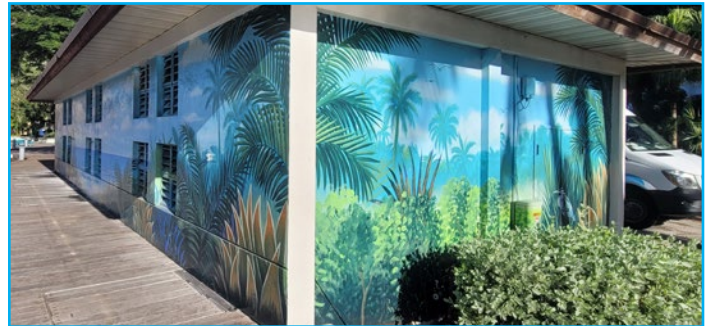
Pump station along Riverwalk
