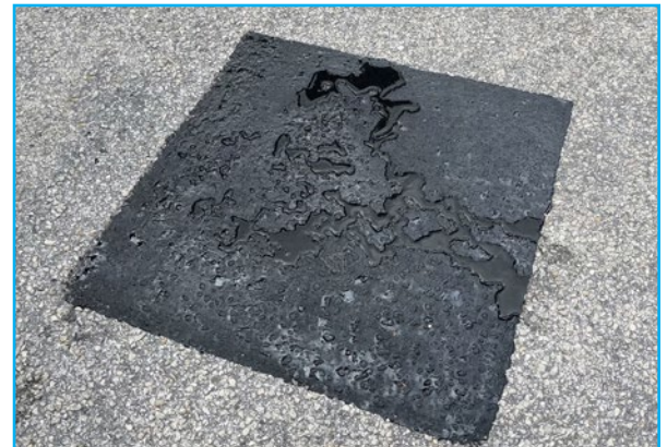
Pothole filled using Road Soup's asphalt repair product
