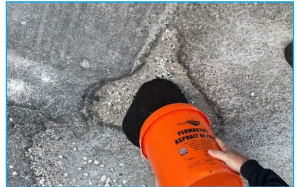
Application of Road Soup's asphalt repair product
