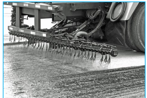
Application of Road Soup's Road Renew product
