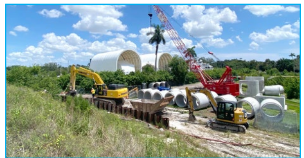
Ongoing stormwater pipe installation near the River Oaks Preserve.
