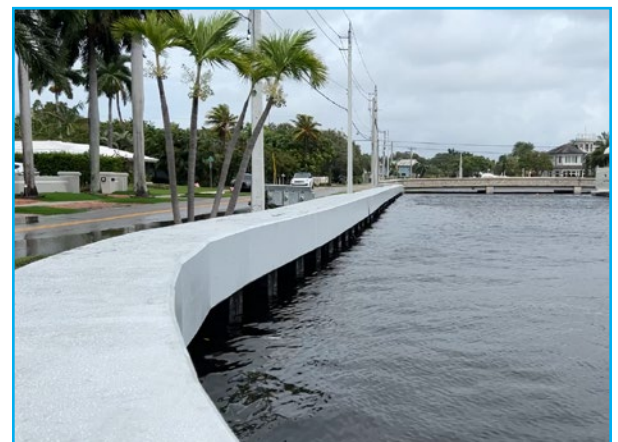
Newly elevated seawall along Cordova Road during Hurricane Ian.
