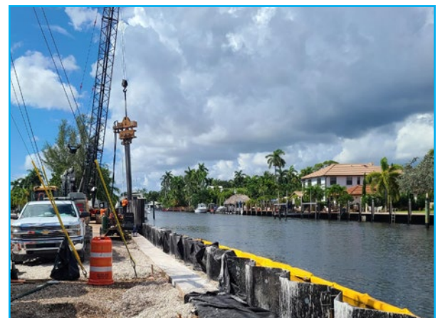
Hendricks Isles seawall under construction.
