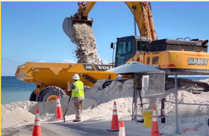
Beach renourishment on Fort Lauderdale Beach
