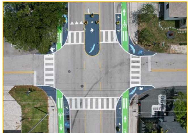
NE 15th Avenue after improvements
