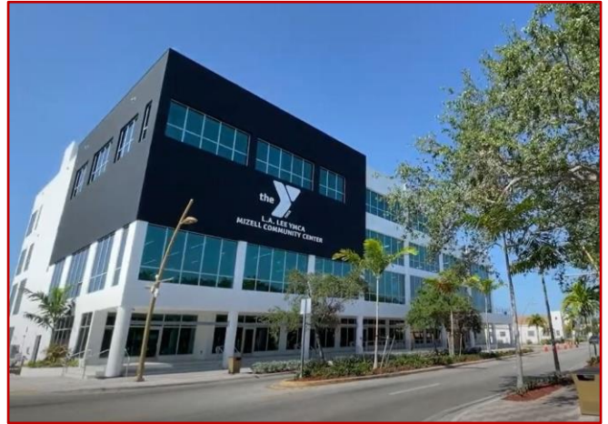
Recently completed LA Lee YMCA/Mizell Community Center
