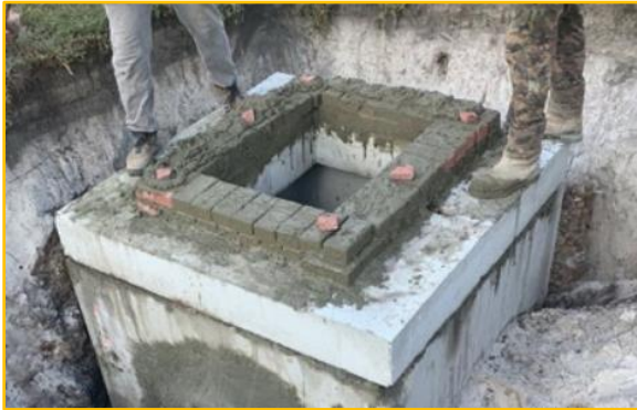
Crews installing a new catch basin in Edgewood
