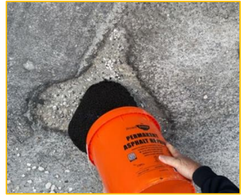
Application of Road Soup's asphalt repair product
