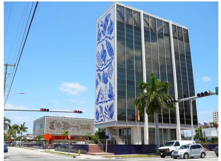
Curtain Wall Construction
