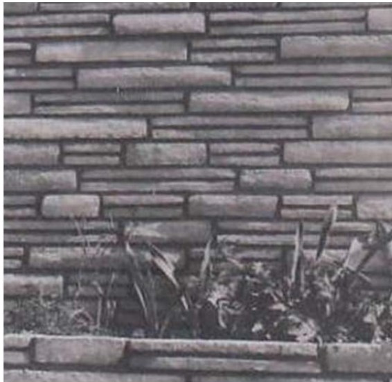
Slumped Brick
