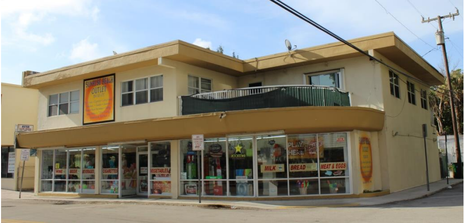
Figure 17: 3100 NE 9 th Street, Sunrise Lane Survey Area (Building #1)
