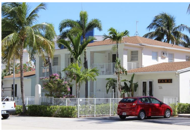
Figure 12: 524 Bayshore Drive, Birch Estates Survey Area (Building #105A)
