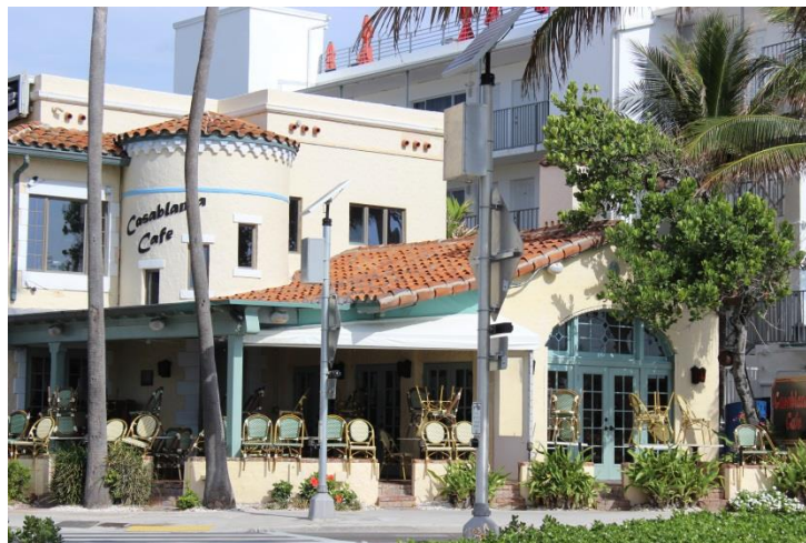
Figure 14: 3029 Alhambra Street, Lauder-Del-Mar Survey Area (Building #8)
