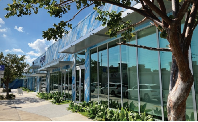
Completion of the Fabrick Project
