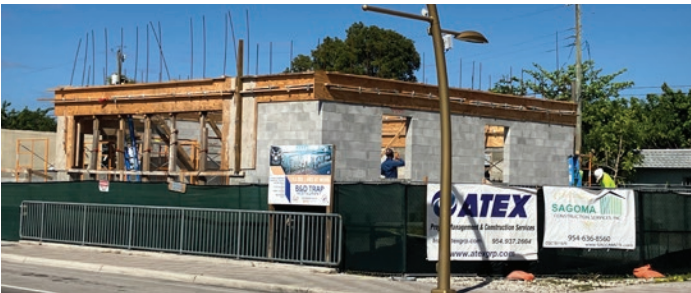
Commencement of construction of B&D Trap Restaurant
