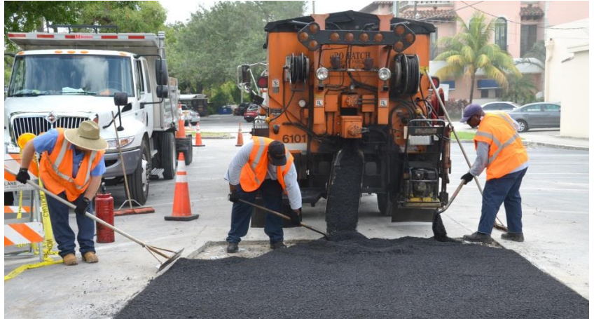
Public Works crew completing hot-in-place asphalt patching
