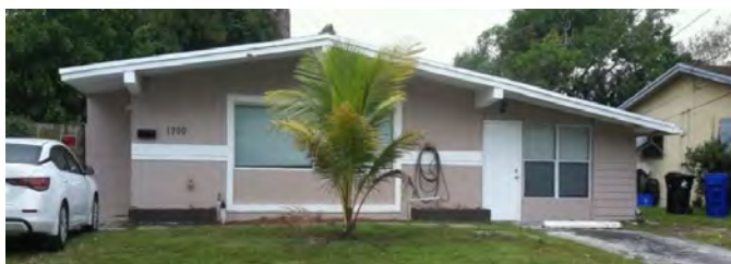
Photos: Representative of the Contemporary style; (1) 1501 SW 9 ST (2) 1700 SW 11 CT
