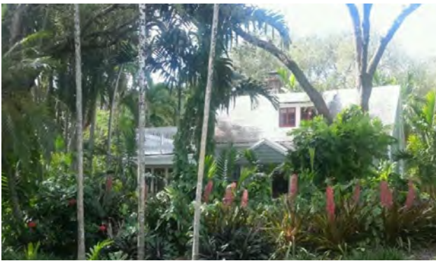
Photos: Representative example of Bungalow style; 701 SW 12th Avenue
