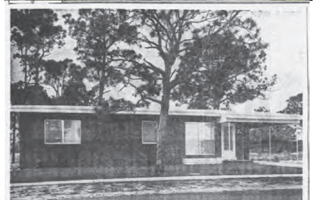
(Daily News photo by Dick Dillon) SHERWOOD FOREST —The lovely home above is one of those recently completed in Sherwood Forest. Address is 1612 SW 10th St. and the new owners are Mr. and Mrs. J. A. Underwood. The sale was handled by Phil Chase, company salesman.
