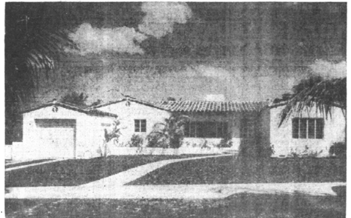
The residence of Mr. and Mrs. Julius Donadt, Rio Vista Blvd., designed by William T. Vaughn, is pictured above. The living room is featured by terrazzo floor and keystone fireplace. Two bedrooms are finished in oak floors. Other rooms include bathroom, dining room, porch, open terrace, kitchen, service porch and bath, including laundry equipment, and garage.
