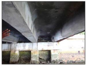
but have the additional problem that they tend to have less load carrying capacity. Once corrosion has started on the reinforcing steel and repeated repairs are needed, section loss to the internal reinforcing steel is very difficult to replace, for the main reason that there is often not enough development length available to splice in new bars and there isn't the space available within the think webs to do so.
