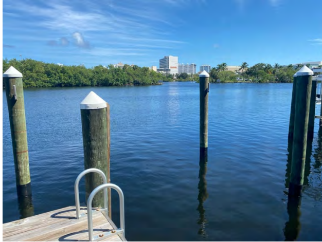
1. Subject site, showing the existing mooring pilings.
