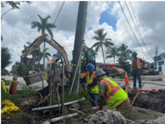
Crews work to underground utility line in the Las Olas Neighborhood
