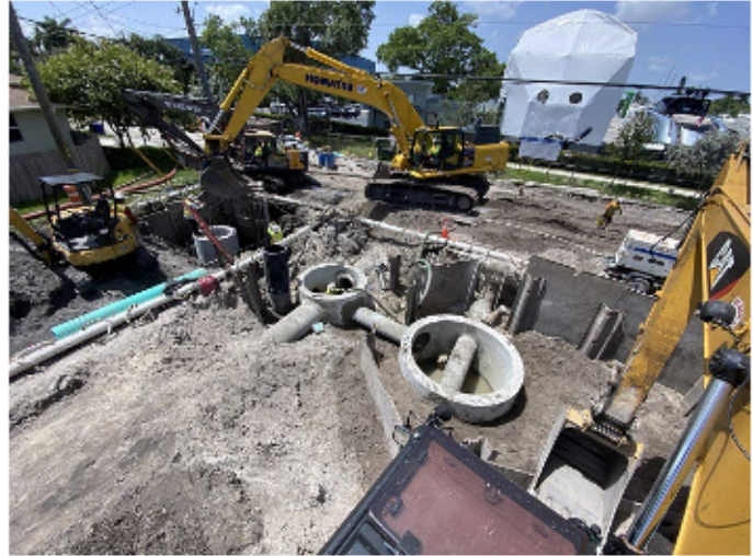
Crews work to construct the River Oaks stormwater pump station
