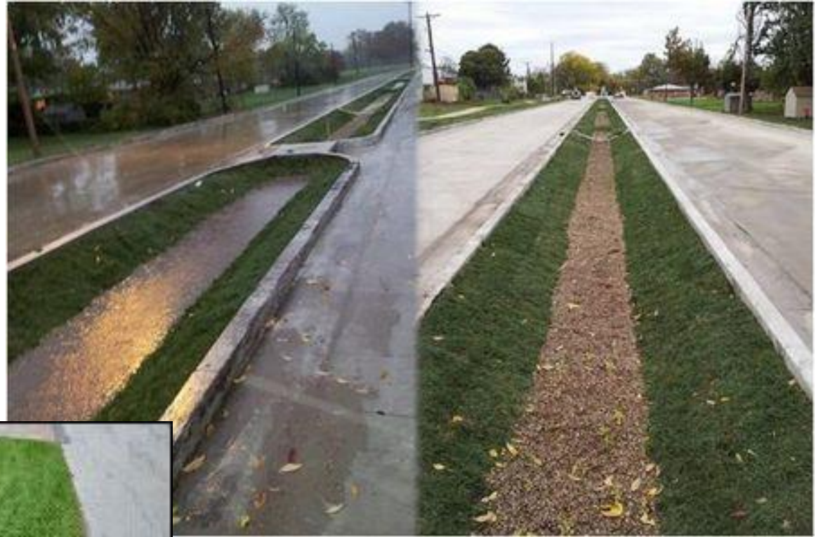
Photo source: Minnesota Stormwater Manual Roadway inversion example
