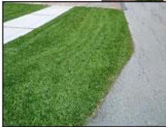
Photo source: City of Ft. Lauderdale Roadside swale example
