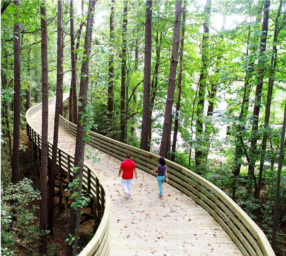
Boardwalk, South Peachtree Creek Greenway, Dekalb County, GA
