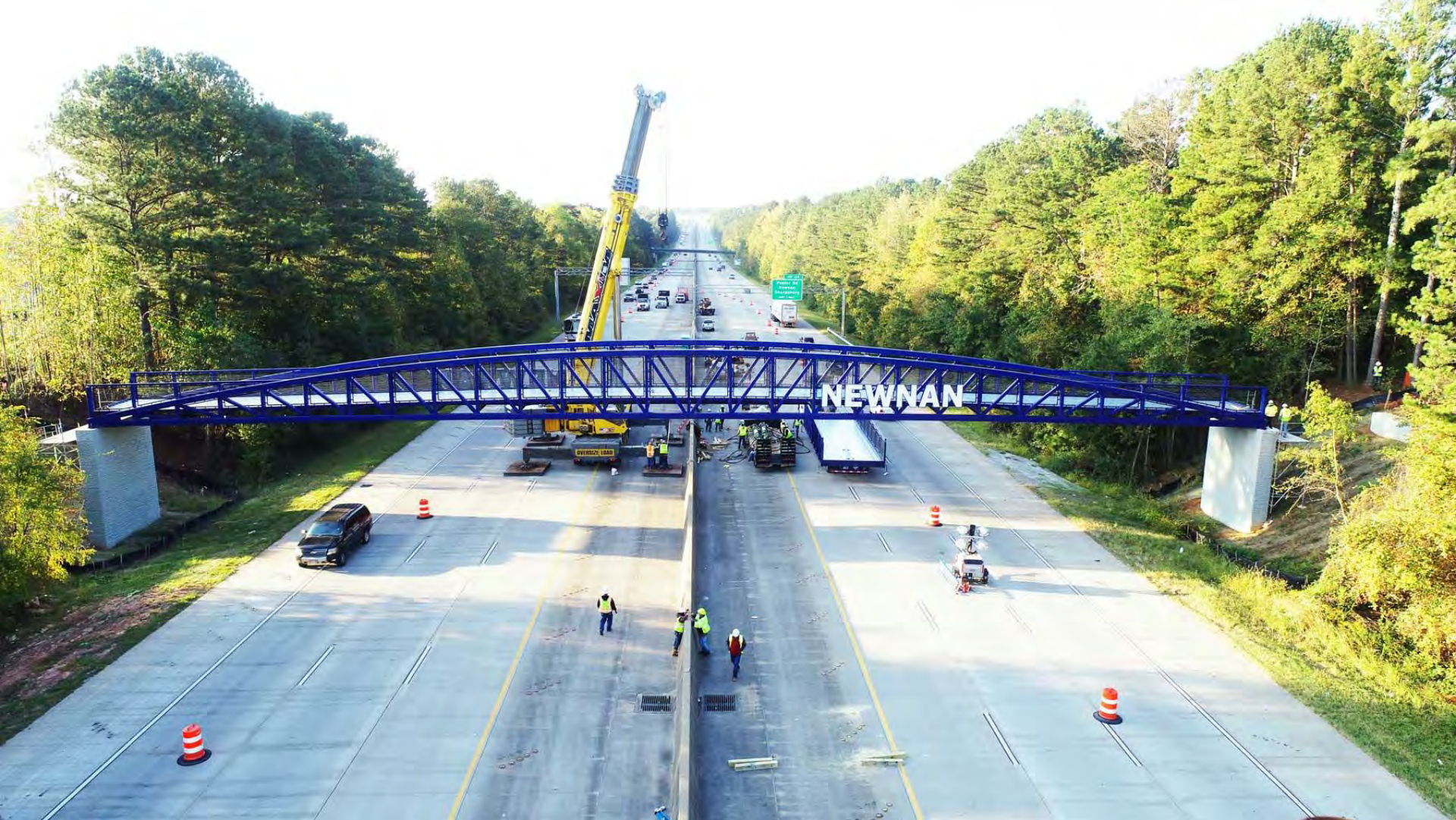
Newnan LINC Bridge over I-85 Newnan, GA
