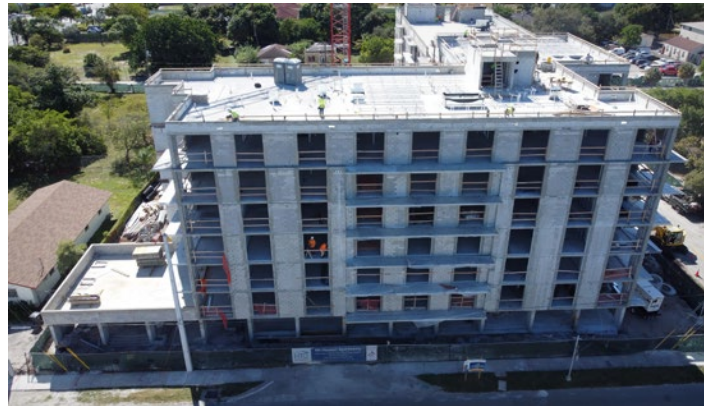
Construction of Mount Hermon Apartments
