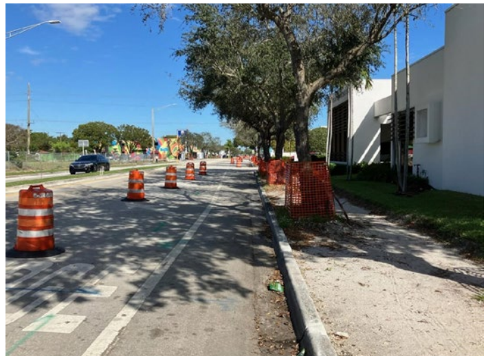
NE 4th Avenue Improvements under Construction
