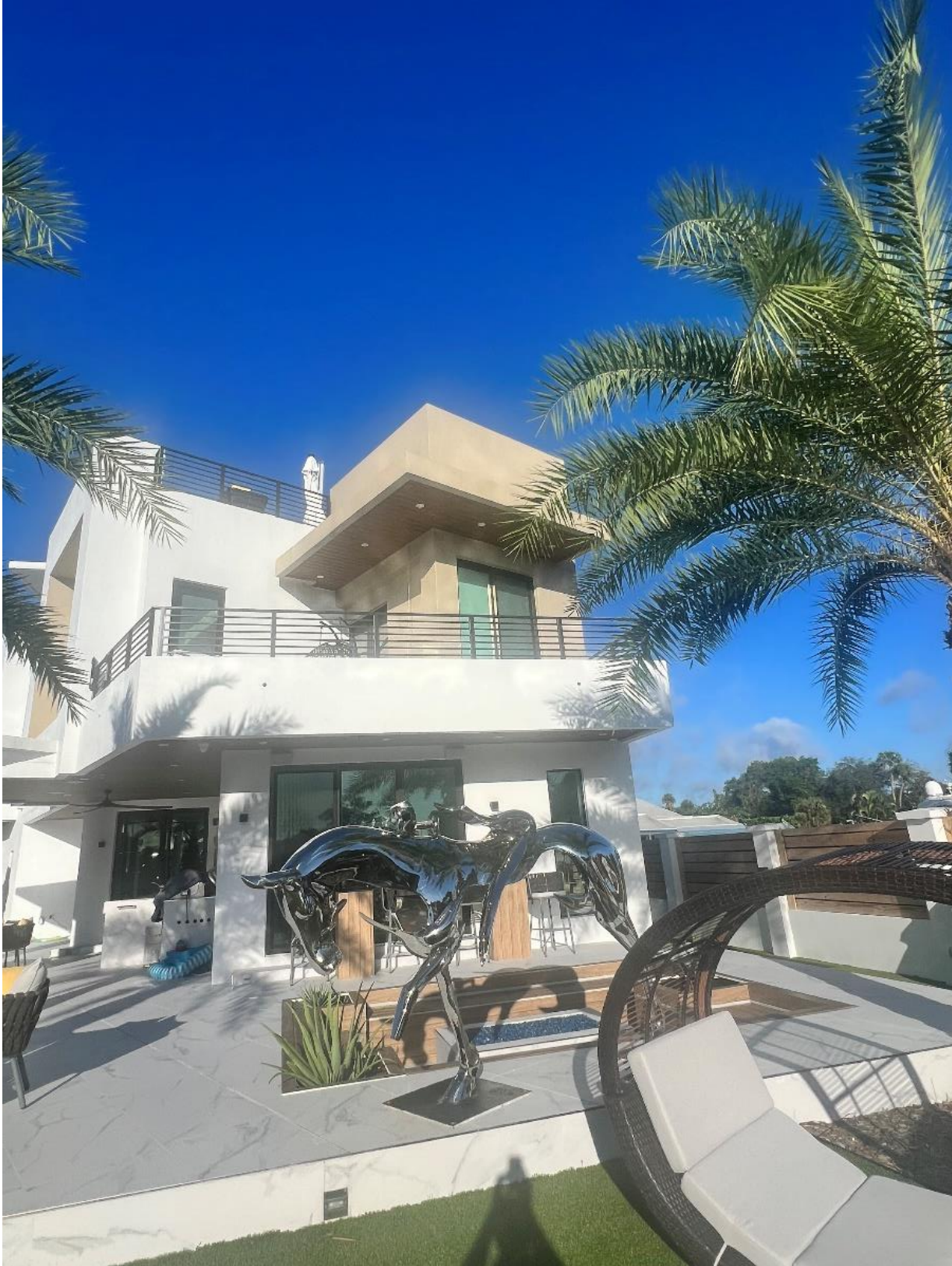
East Rear / Side Yard Area Facing West
