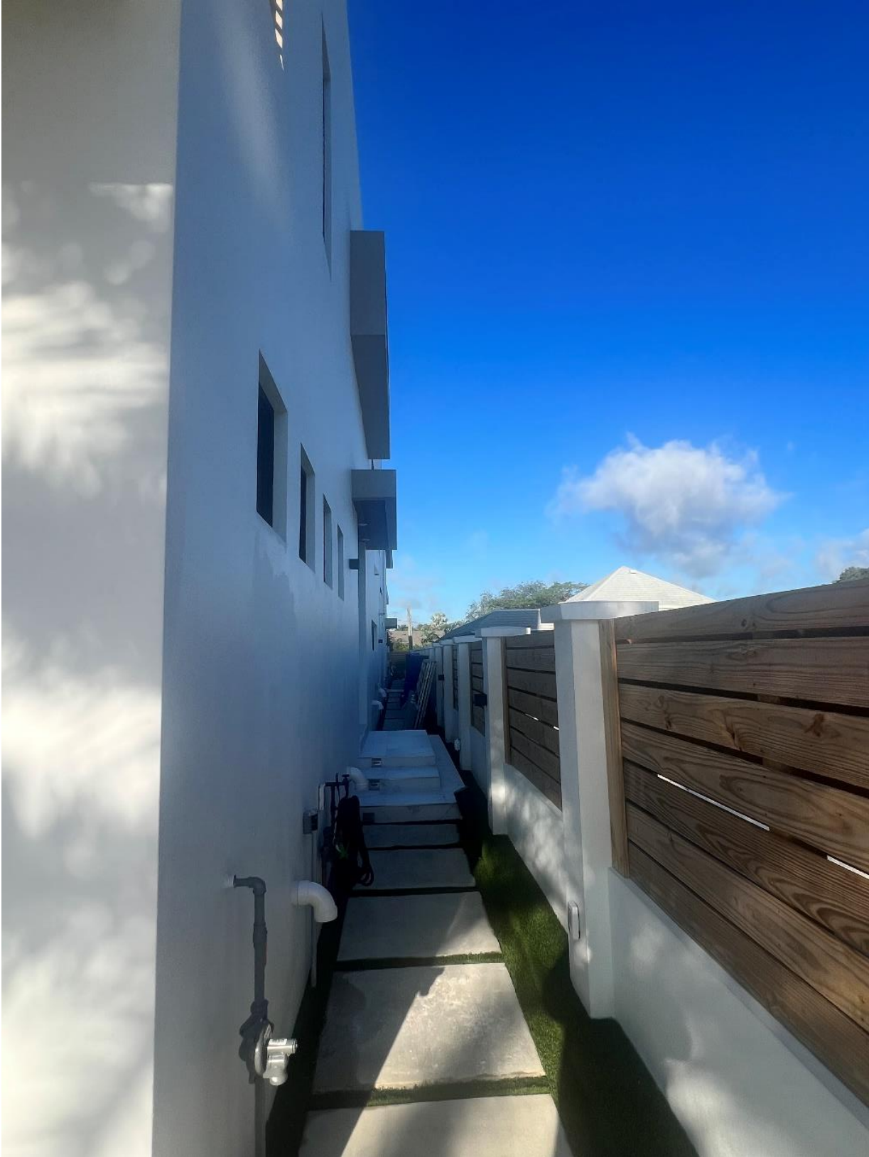
Side Yard Area facing towards the West
