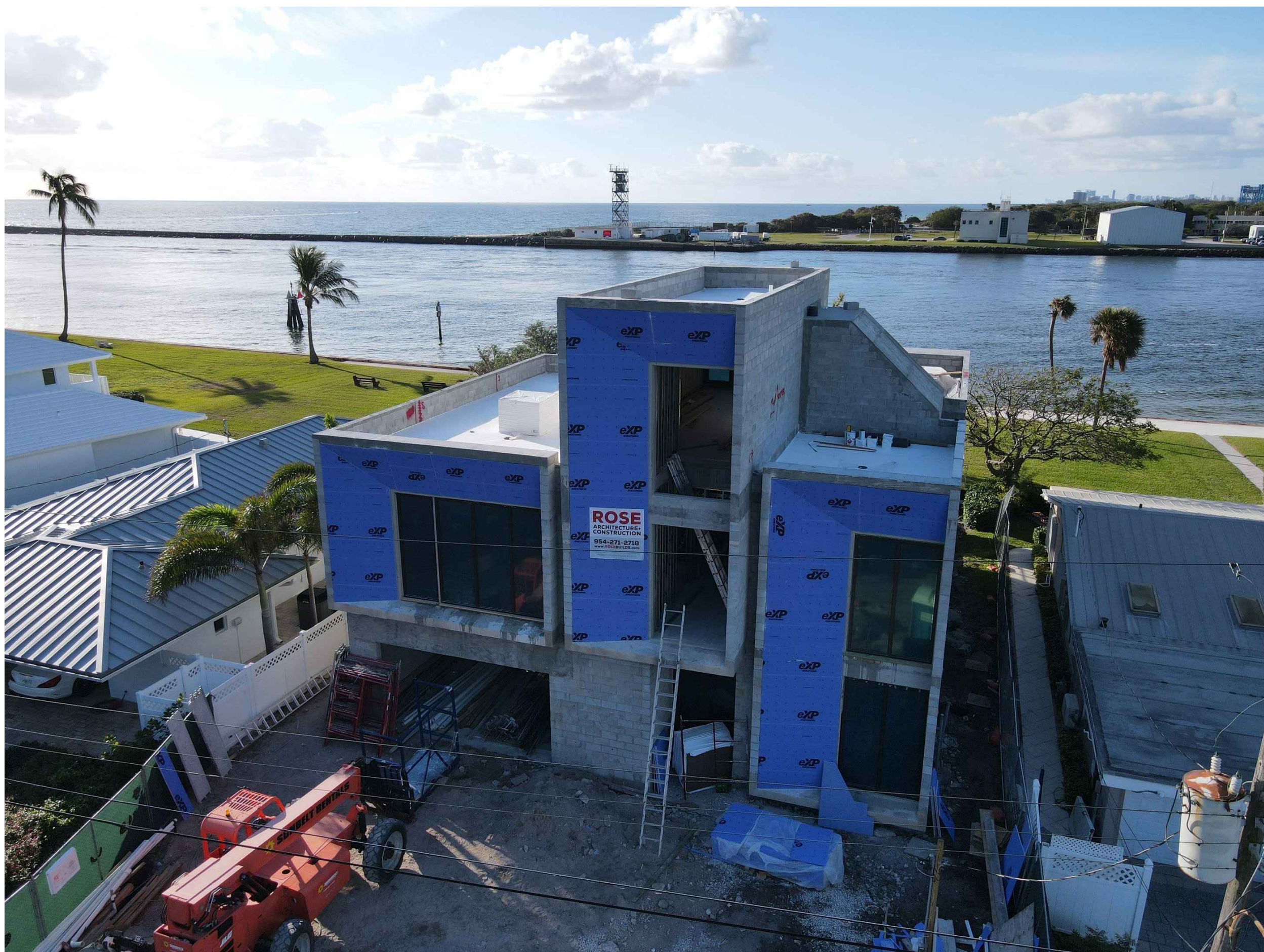
PHOTO #2: NORTH - EAST AERIAL VIEW (UNDER CONSTRUCTION)
