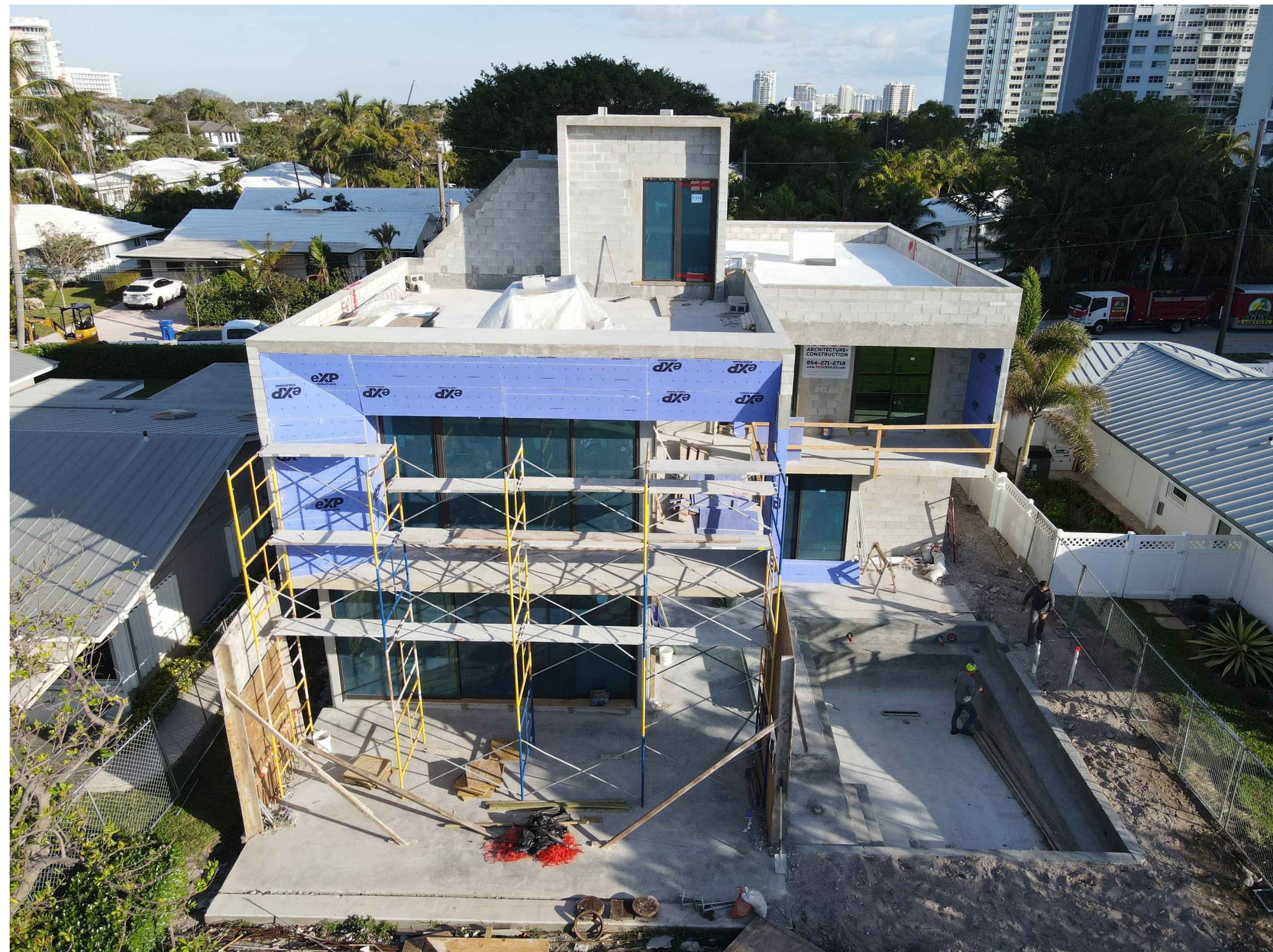
PHOTO #4: SOUTH AERIAL VIEW (UNDER CONSTRUCTION)
