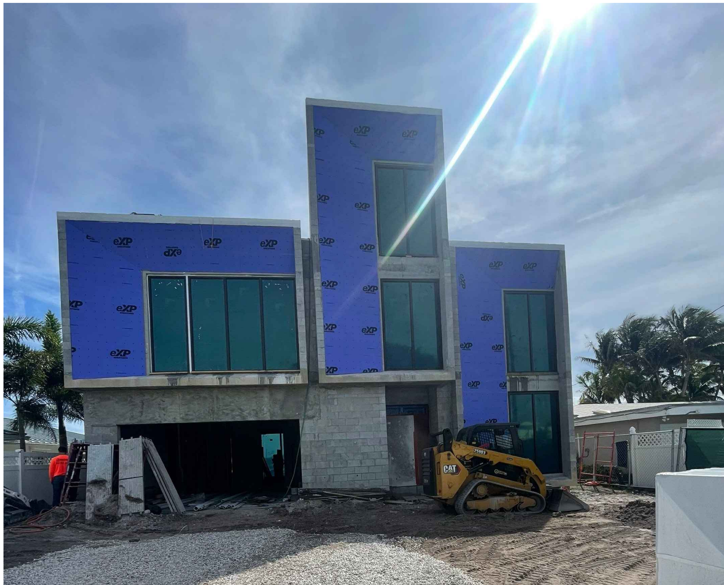
PHOTO #1: NORTH VIEW (UNDER CONSTRUCTION)
