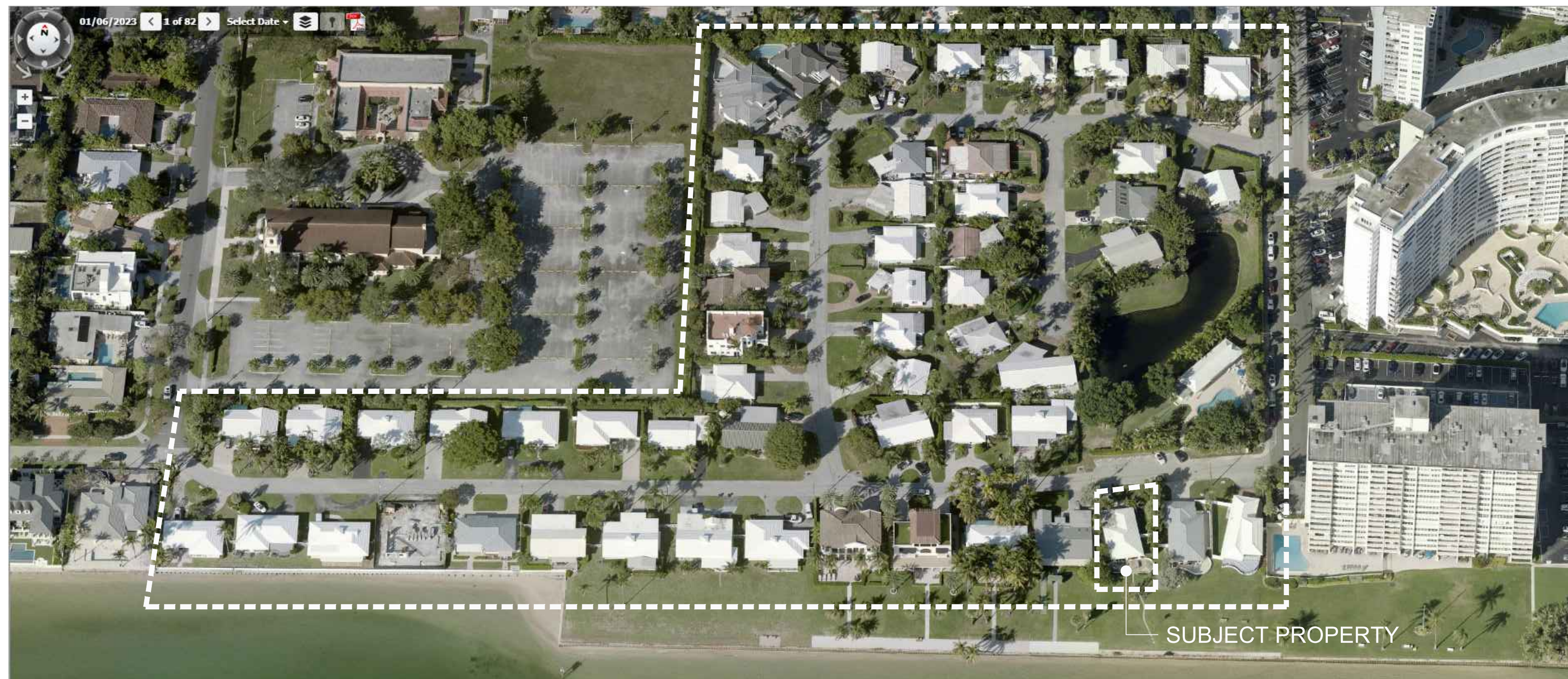
PHOTO #6: BREAKWATER AERIAL SOUTH
