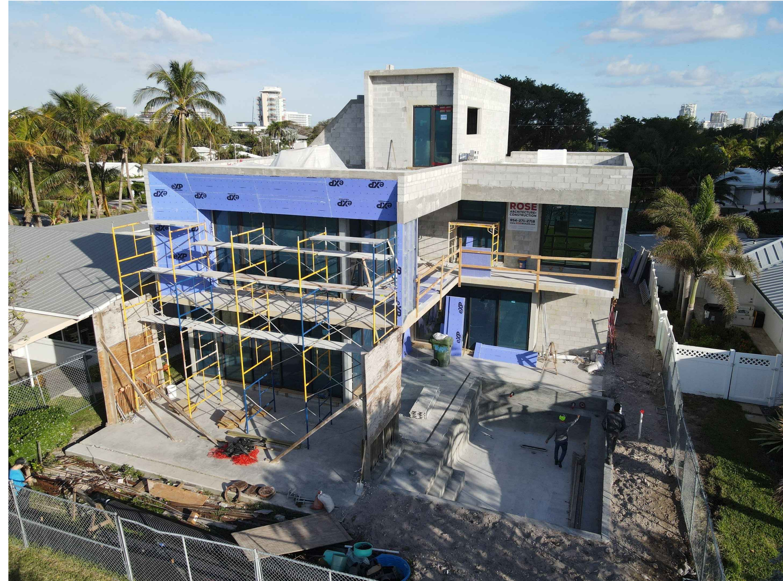
PHOTO #5: SOUTH – WEST AERIAL VIEW (UNDER CONSTRUCTION)
