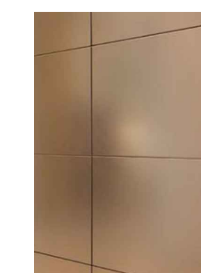
G ALUM. CLADDING BRONZE METAL FINISH
