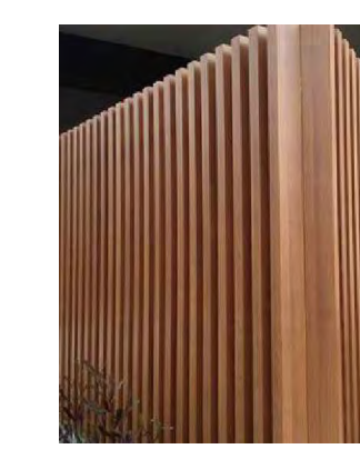
F 2" X 4" ALUM. SCREEN, 50% TRANSPARENCY WOODEN FINISH
