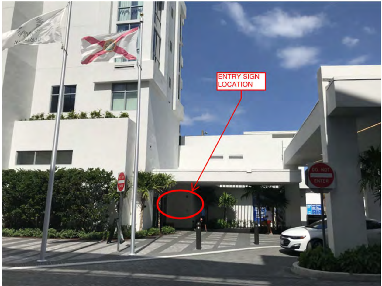
West side of Hotel/Retail building. Porte cochere on the right. The entry is to the right of the State of Florida flag pole, and almost impossible to identify.
