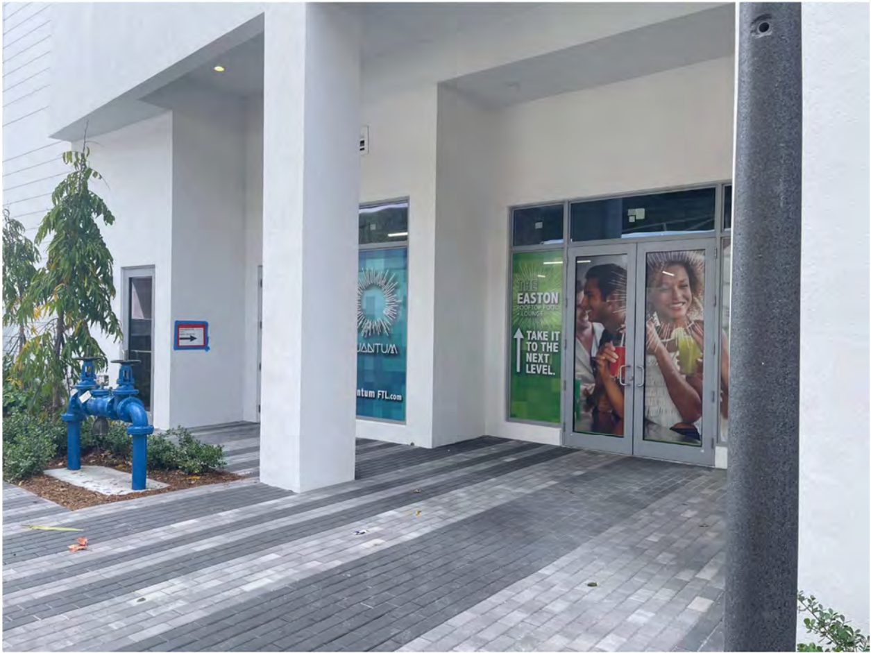
The Easton entry is the door on the left. Note the overhang over it is very small. A canopy is needed. Also, note the other door and windows you see here are recessed deeper into the building, and they belong to a different business.
