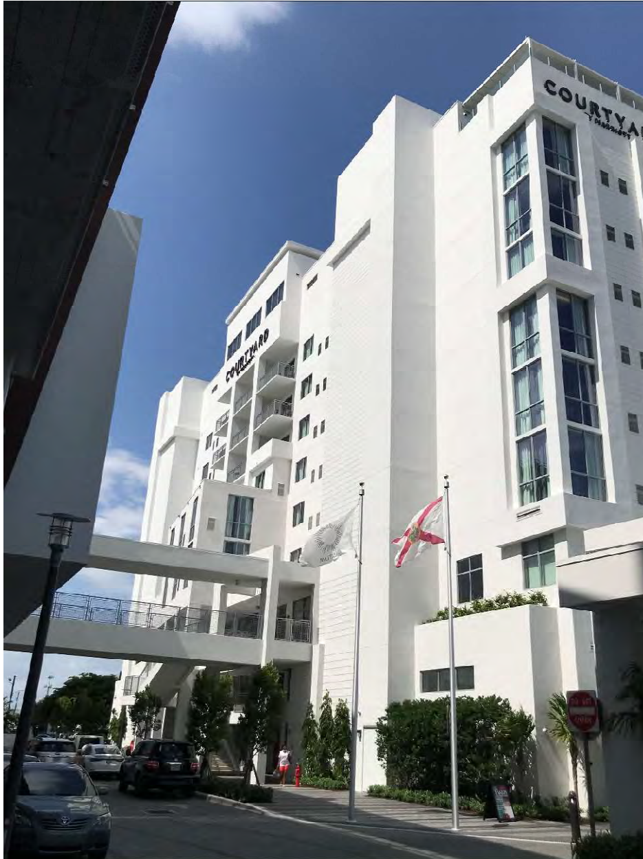
West side of Hotel/Retail building (retail on first floor and hotel above it). Standing on 5 th Tr. looking northeast, and north of previous location. Existing “Courtyard” sign at the top of the west side of the building (sign 2). Also visible is the “Courtyard” sign (sign 1) on the south side, from the previous photograph.
