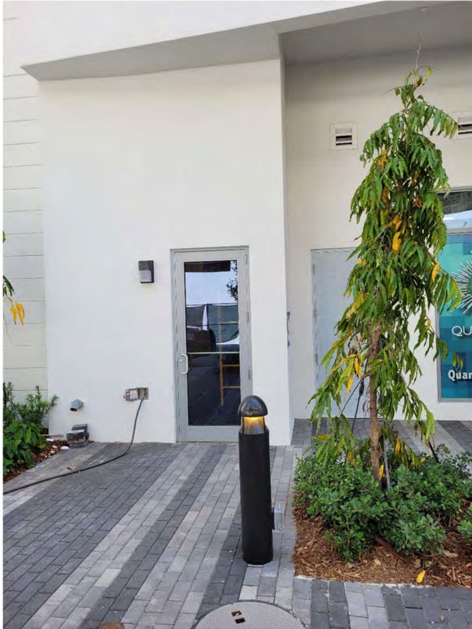
The Easton entry is the door on the left. Note the overhang over it is very small. A canopy is needed. Also, note the other door and window you see here are recessed deeper into the building, and they belong to a different business.
