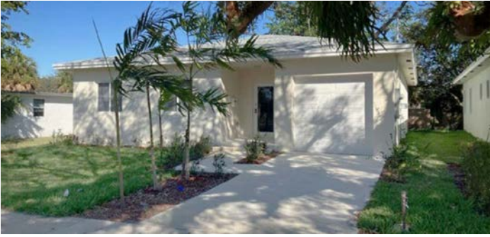
Scattered Site Infill Housing in Durrs Neighborhood - Lemon City Development
