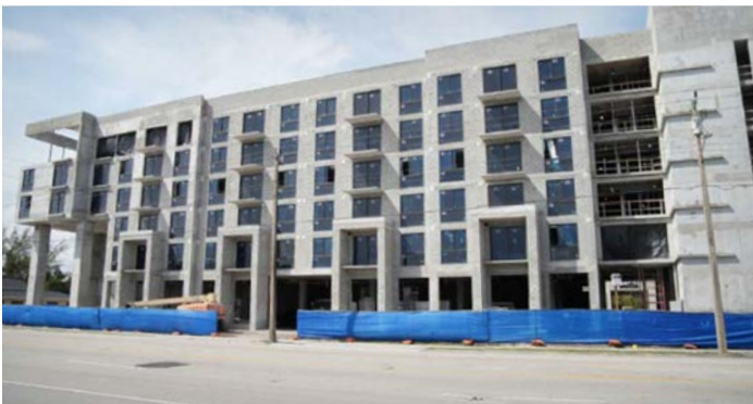
Construction of the The Adderley
