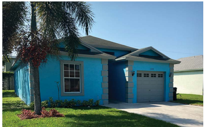
CRA Façade and Landscaping Program Improvements in the Durrs Neighborhood
