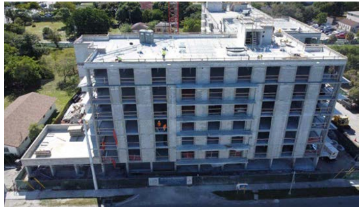
Construction of Mount Hermon Apartments
