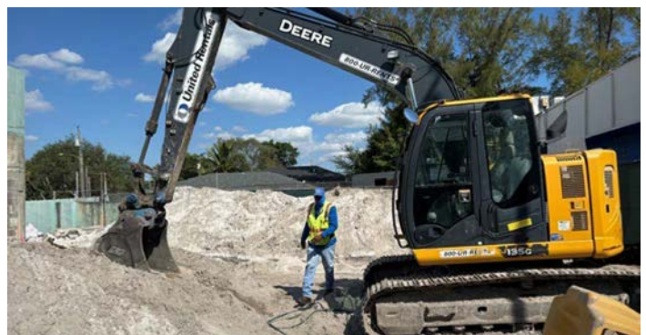
Construction of new American Legion Robert Bethel Post 220
