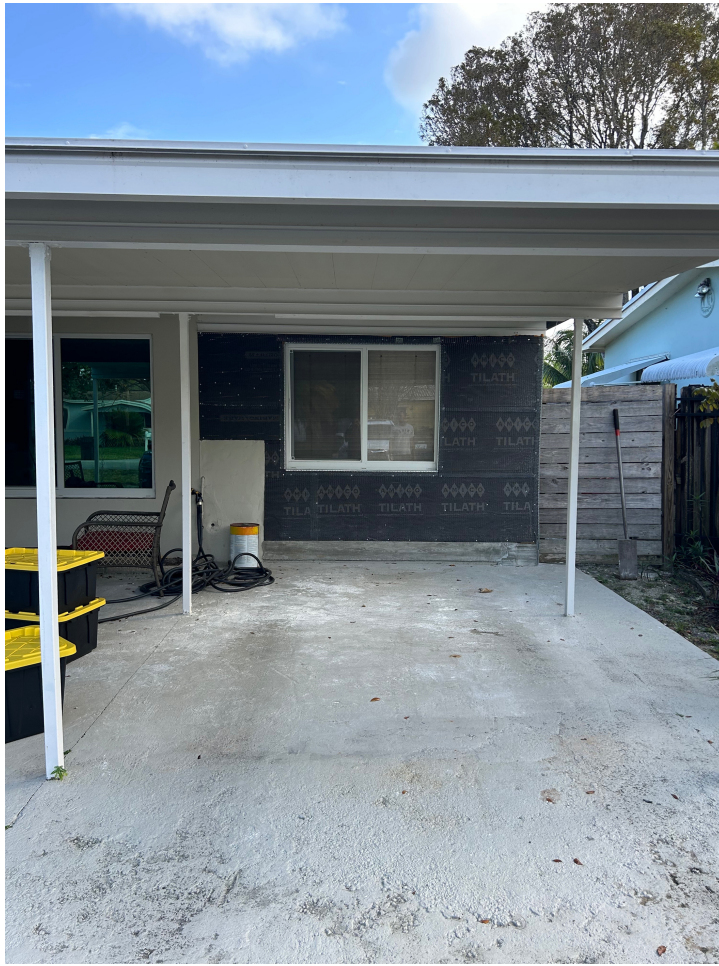
#7 Front street view of structure north facing
