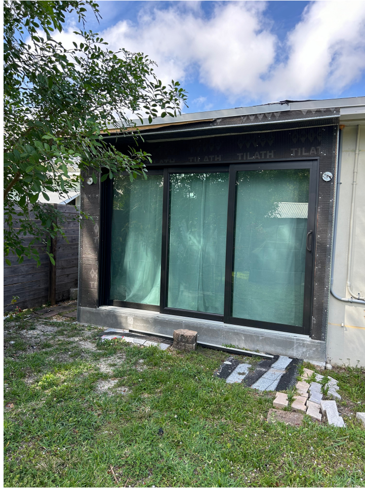
#4 Backyard view of structure facing south
