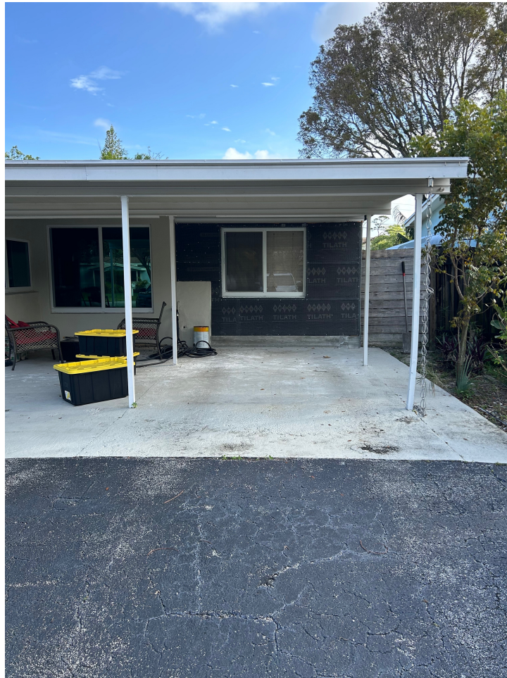
#6 Front street view of structure north facing
