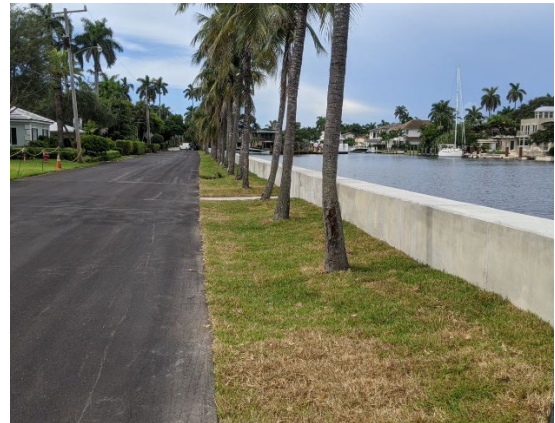
Isles of Palms Sewall after improvements
