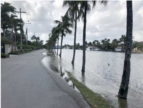
Isles of Palms Sewall before improvements
