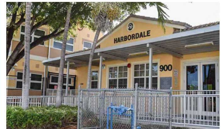
Harbordale Elementary School
