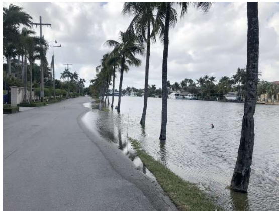
Isles of Palms Seawall before improvements
