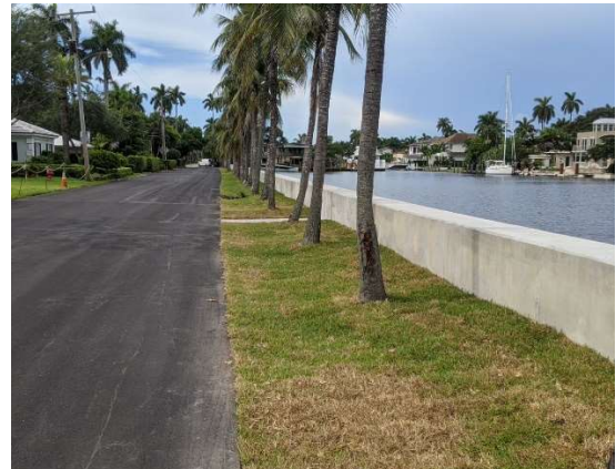
Isles of Palms Seawall after improvements
