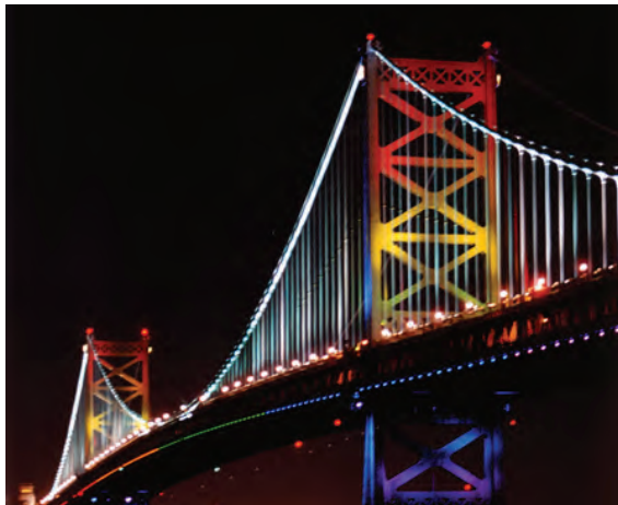
Ben Franklin Bridge Philadelphia
