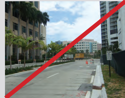
Pavement does not need to be this wide.
