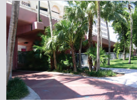
Andrews Bridge Before
