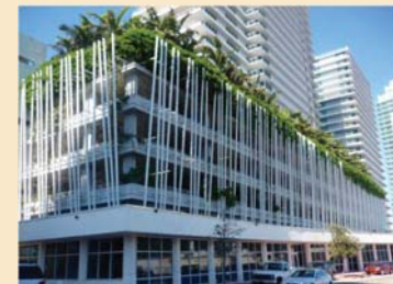
[Figure 4.254] A parking garage with sophisticated styling, screening, windows and green roof elements integrated into the design.
