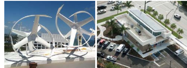
[Figures 4.266 & 4.267] Left: Wind turbines on top of a hotel at Fort Lauderdale beach. Right: a LEED Certified bank near Downtown Fort Lauderdale.
